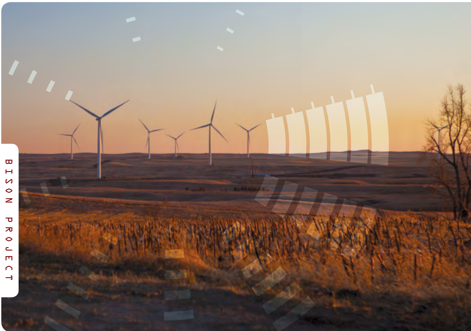
A RELATIVELY SNOW-FREE WINTER IN SOUTH-CENTRAL NORTH DAKOTA ALLOWED MUCH PROGRESS ON THE ACCELERATED SECOND AND THIRD PHASES OF THE BISON WIND ENERGY CENTER. BY THE END OF 2011, MORE THAN HALF THE TURBINE AND SUBSTATION FOUNDATIONS WERE COMPLETED ON BISON 2, WITH NEARLY ALL TURBINE ACCESS ROADS FINISHED. THE WIND FARM WILL GROW FROM 31 TURBINES TO 101 TURBINES IN 2012.
